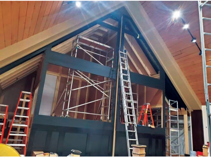
Photo 8: Structure during installation
