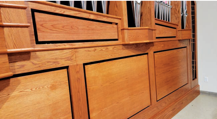
Photo 9: Case panels allowing tonal egress for bass
