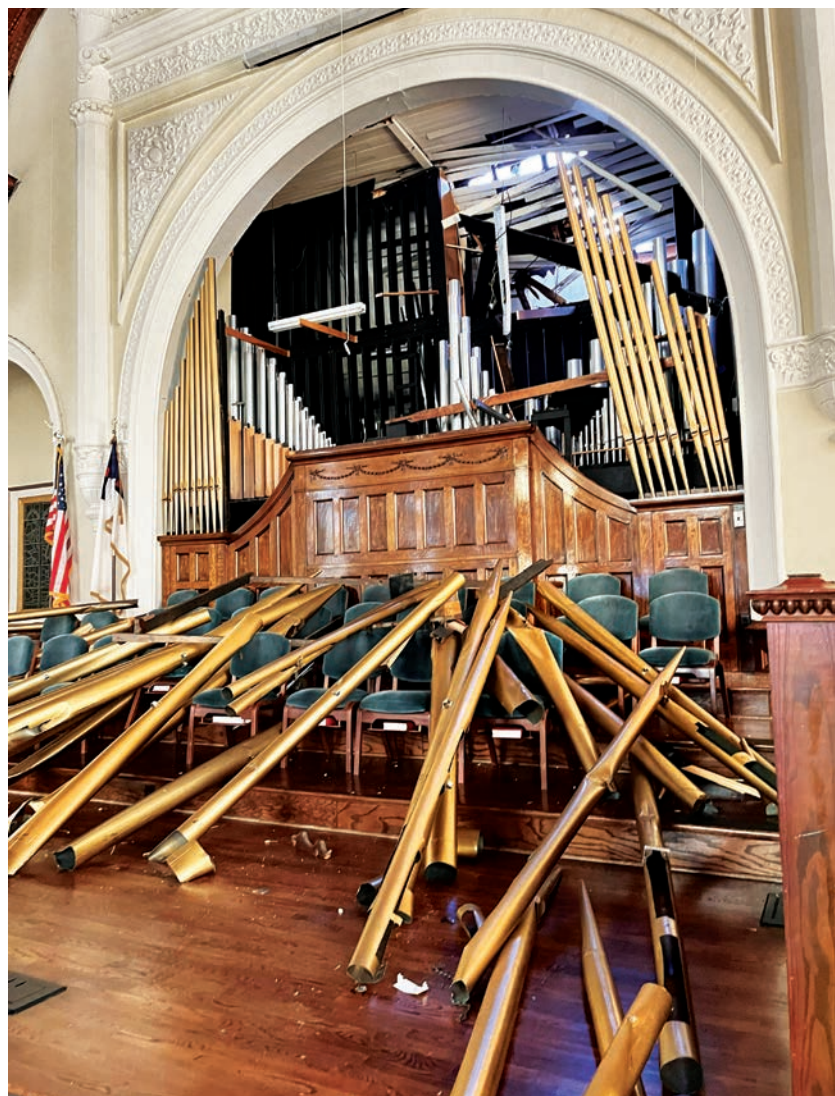
Close-up of damage to organ and façade from collapsing chimney
