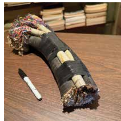
Console cable, Trinity Church, Boston, Massachusetts (photo credit: John Bishop)
