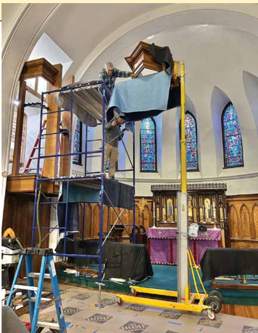
Bart Dahlstrom and Dave Mitchell assist in raising the last piece of the organ case—the crown on the center tower—during the organ's installation in March 2025
