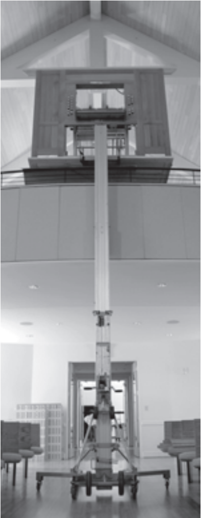
Lifting the console over the balcony rail
