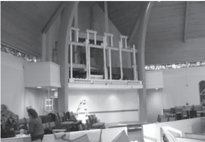
Support racking in place awaiting the 16' Principals
