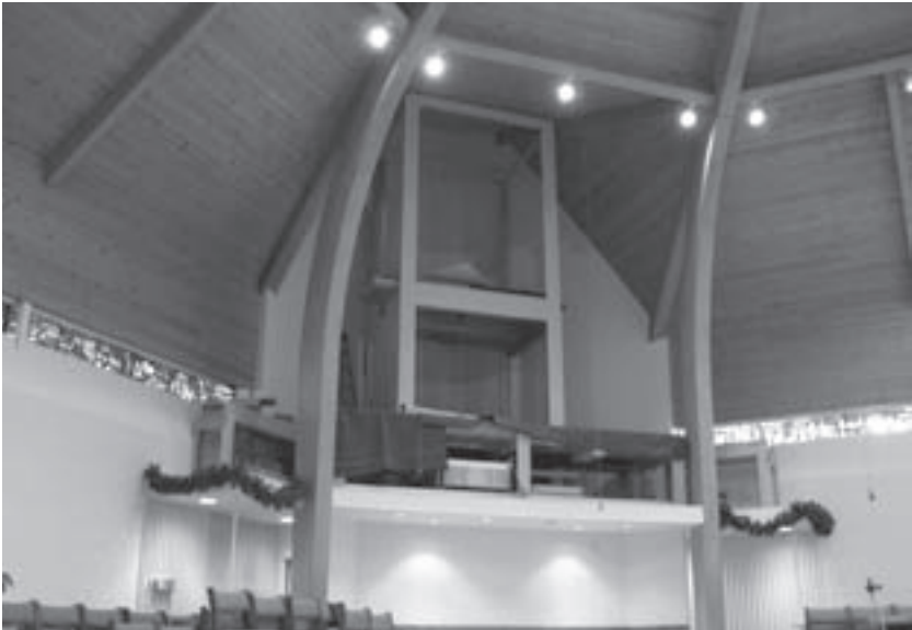
Early installation: windchests and Swell and Choir boxes
